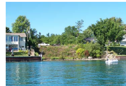
A natural shoreline can be seen here in Marysville located between two engineered seawalls.
